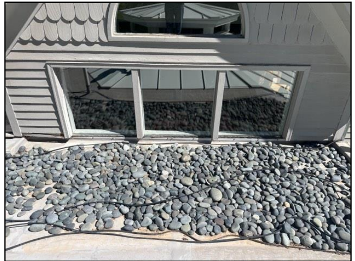
Inadequate sill projection
