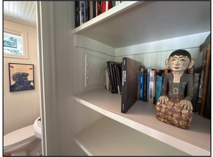
Panel is painted/caulked to wall. Removing...
