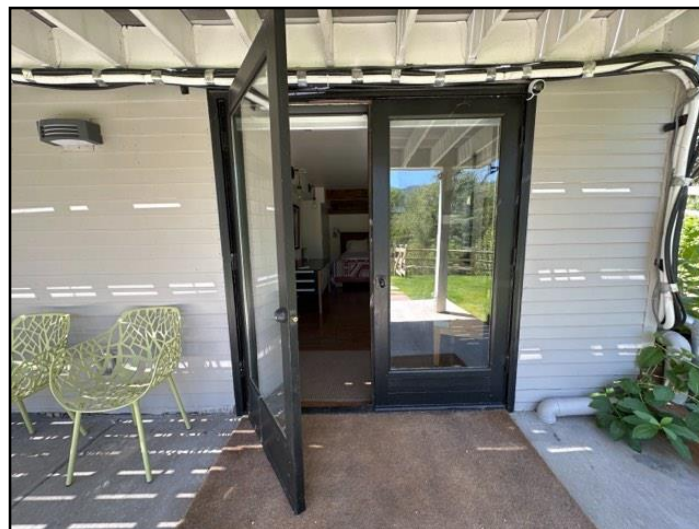
Installed backwards
