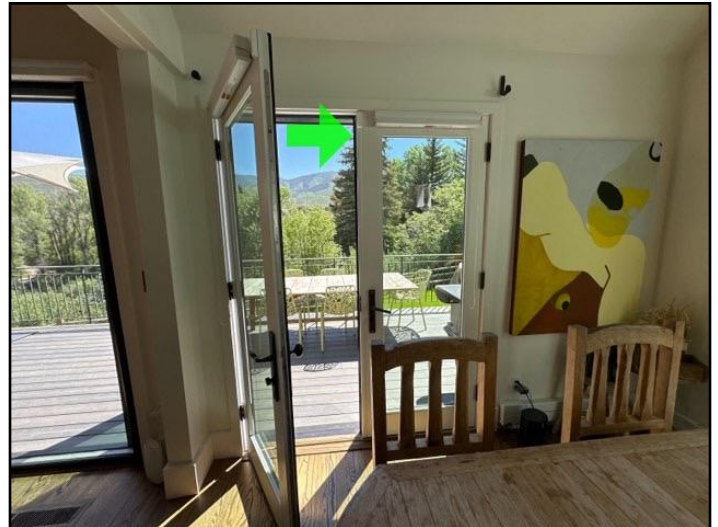
Missing or damaged
