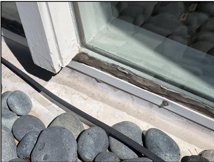
Inadequate sill projection
