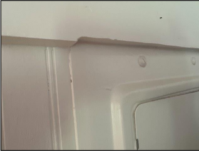
Panel is painted/caulked to wall. Removing...
